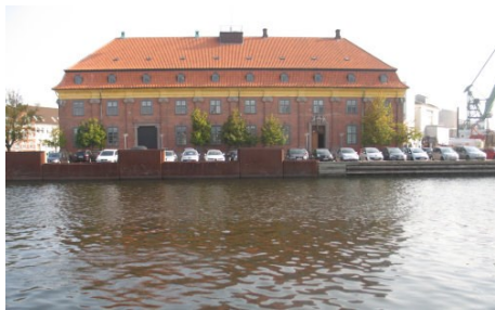
Toldbodens facade mod vest
