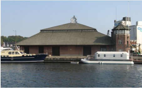
Stykgodspakhusets facade mod vest
